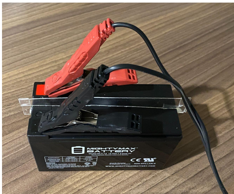
(Figure 18: Picture of 12V battery being charged)
